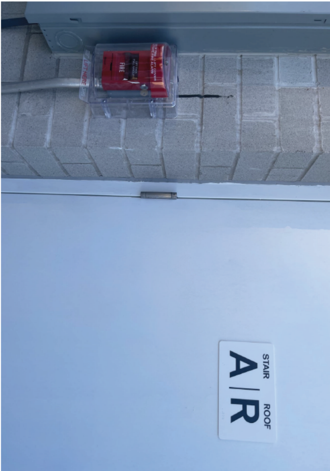
WEATHER PROTECTED COVERING FOR OUTDOOR PULL STATIONS
