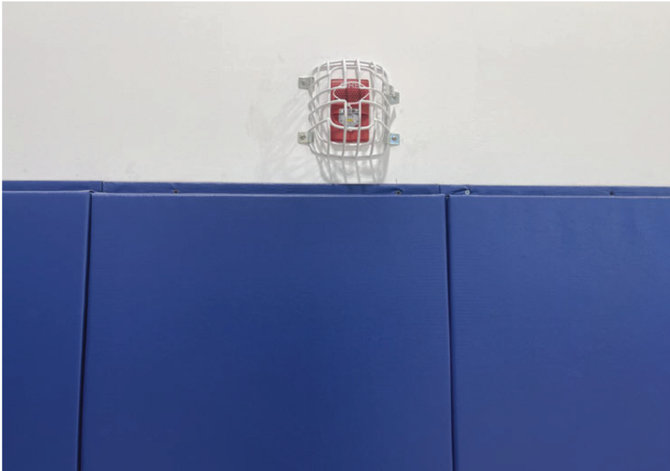
PROTECTED CAGES FOR FIRE ALARM STROBES
