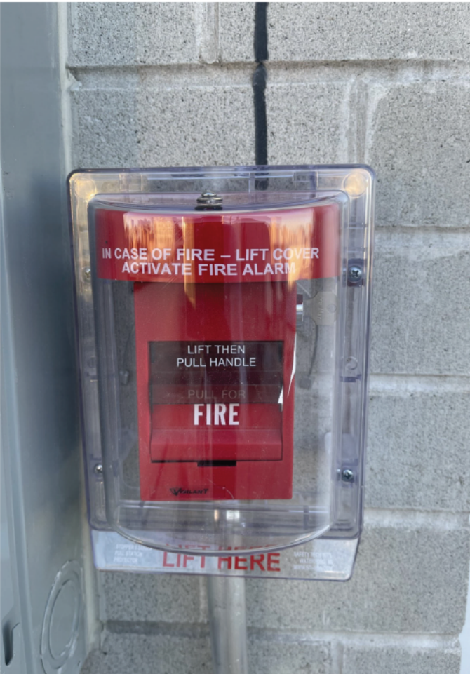
WEATHER PROTECTED COVERING FOR OUTDOOR PULL STATIONS
